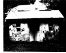
268 - Sweeneys Cottage Eltham 12 - Shire of Eltham Heritage Study 1992
