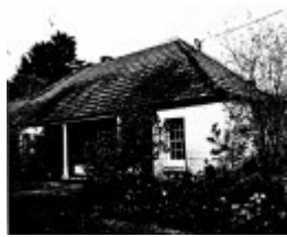
268 - Sweeneys Cottage Eltham 02 - Shire of Eltham Heritage Study 1992
