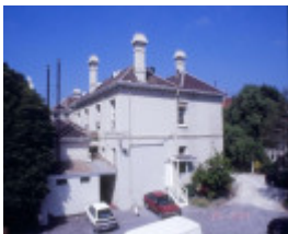
h01619 airlie domain road south yarra rear main bldg she project 2004
