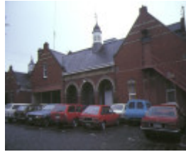
H01619 airlie domain road south yarra police officers college former stable at rear
