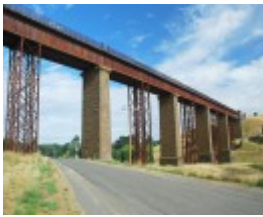
TARADALE RAILWAY PRECINCT (MURRAY VALLEY RAILWAY, MELBOURNE TO ECHUCA) SOHE 2008
