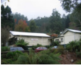
side of building
