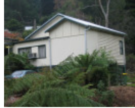
rear of building
