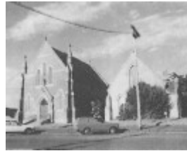
Former Wesleyan Churches, 79 -81 Hesse Street, Queenscliff
