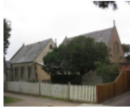
Former Wesleyan Churches, 79 -81 Hesse Street, Queenscliff
