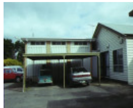
kardinia house riverview terrace belmont additions
