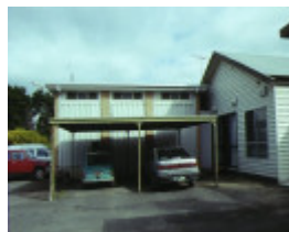
kardinia house riverview terrace belmont additions
