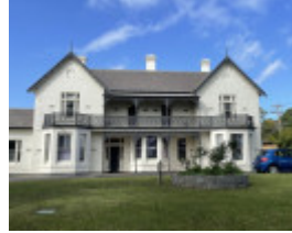
Kardinia House primary facade. 2023.
