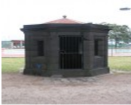
TIDE GAUGE HOUSE SOHE 2008
