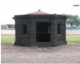
TIDE GAUGE HOUSE SOHE 2008
