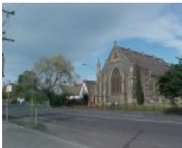
H00633 1 former st giles church and free church school geelong oct01
