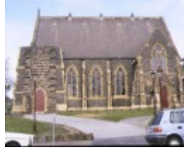
St Giles Church Geelong Church Front View
