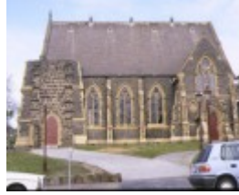
St Giles Church Geelong Church Front View
