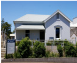
H543 orderly room residence
