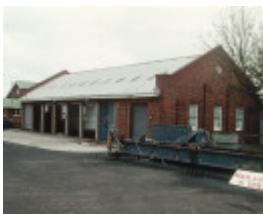
H01098 rafa barracks gun shed 1995
