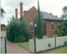
h01098 rafa barracks single men s quarters 2002
