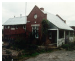
H01098 rafa barracks horse hospital demolished 1995
