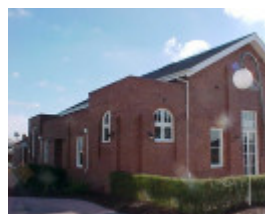
H01098 rafa barracks gymnasium 2001 pm1
