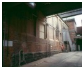
h02050 richmond maltings east elevation 1880 malthouse mz june03
