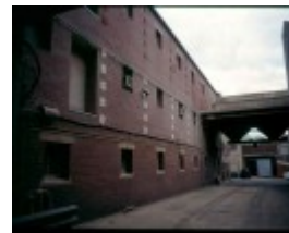
h02050 richmond maltings west elevation 1930 malthouse mz jun03
