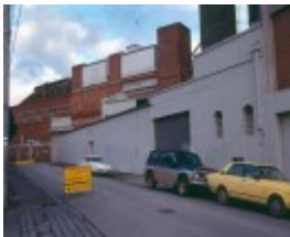
h02050 richmond maltings view east along gough st ro june03
