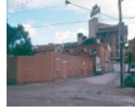
h02050 1 richmond maltings view along gough st ro jun03
