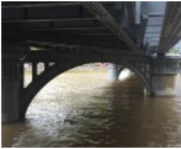
SANDRIDGE RAILWAY LINE BRIDGE October 2016
