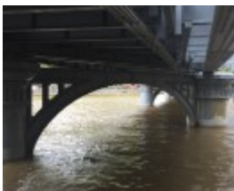
SANDRIDGE RAILWAY LINE BRIDGE October 2016
