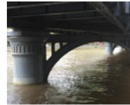
SANDRIDGE RAILWAY LINE BRIDGE October 2016
