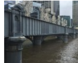
SANDRIDGE RAILWAY LINE BRIDGE October 2016
