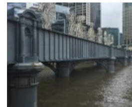
SANDRIDGE RAILWAY LINE BRIDGE October 2016
