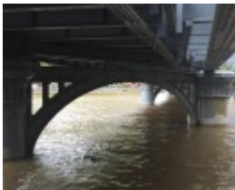
SANDRIDGE RAILWAY LINE BRIDGE October 2016
