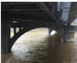
SANDRIDGE RAILWAY LINE BRIDGE October 2016
