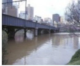
1 sandridge railway line bridge over yarra river melbourne view over river aug1985
