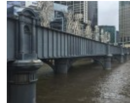
SANDRIDGE RAILWAY LINE BRIDGE October 2016
