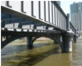
SANDRIDGE RAILWAY LINE BRIDGE SOHE 2008
