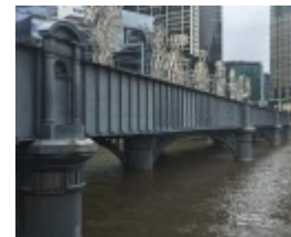
SANDRIDGE RAILWAY LINE BRIDGE October 2016
