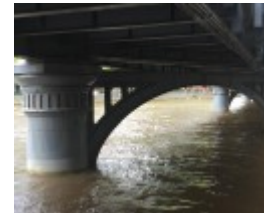
SANDRIDGE RAILWAY LINE BRIDGE October 2016
