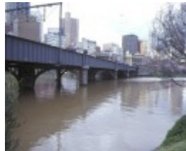
1 sandridge railway line bridge over yarra river melbourne view over river aug1985
