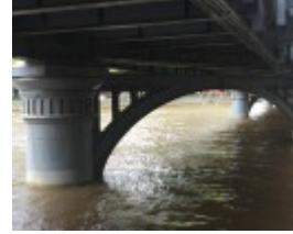
SANDRIDGE RAILWAY LINE BRIDGE October 2016
