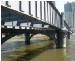
SANDRIDGE RAILWAY LINE BRIDGE SOHE 2008
