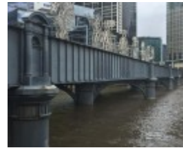
SANDRIDGE RAILWAY LINE BRIDGE October 2016
