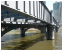
SANDRIDGE RAILWAY LINE BRIDGE SOHE 2008
