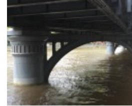
SANDRIDGE RAILWAY LINE BRIDGE October 2016
