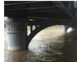
SANDRIDGE RAILWAY LINE BRIDGE October 2016
