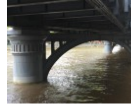
SANDRIDGE RAILWAY LINE BRIDGE October 2016
