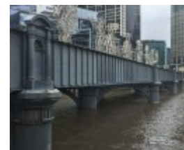
SANDRIDGE RAILWAY LINE BRIDGE October 2016
