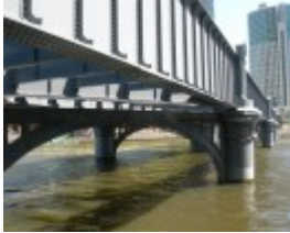
SANDRIDGE RAILWAY LINE BRIDGE SOHE 2008
