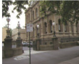
law courts bendigo entrance gates jan1999
