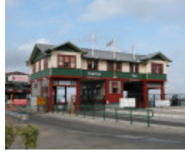
Station Pier Port Melbourne July 2003 Gatehouse
