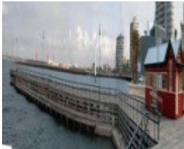
Station Pier Port Melbourne July 2003 West Wing And Shed
