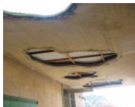
Maribyrnong substation cutouts in concrete roof
