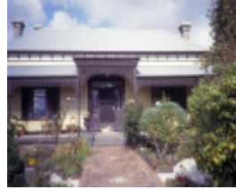
h01168 1 yarrowee hall darling street ballarat facade of house she project 2003
