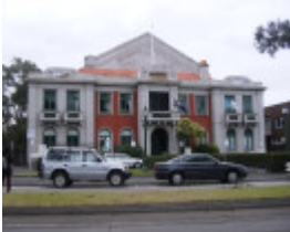
City of Williamstown Municipal Offices and Town Hall (former) and Drinking Fountain, Hobsons Bay Heritage Study 2006
