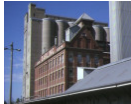
john darling & son flour mill albion silos
