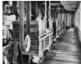
c 1948 copy of negative of an image showing the John Darling Flour Mill's pan-sifter floor
