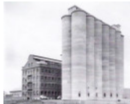
c 1940 depicting the south-west facade of the complex including the 1926-7 storehouse and mill building and the 1939 reinforced concrete silos
