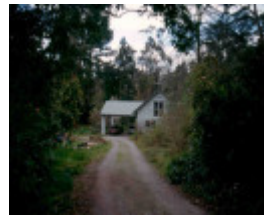
h02053 h2053 bv spinney 15 bv road june 2003
