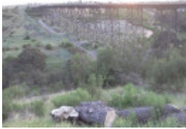
B5235 Albion Viaduct
