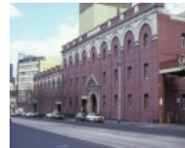
carlton brewery external front swanston street
