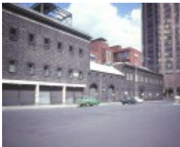
carlton brewery bouverie street carlton side view
