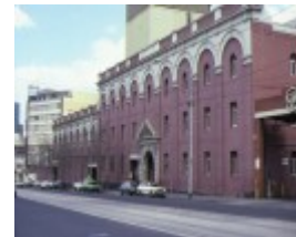
carlton brewery external front swanston street
