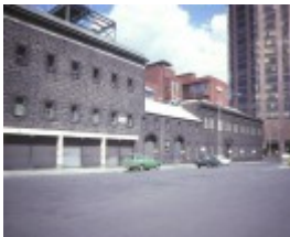
carlton brewery bouverie street carlton side view
