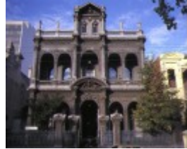
1 benvuta drummond street carlton front view
