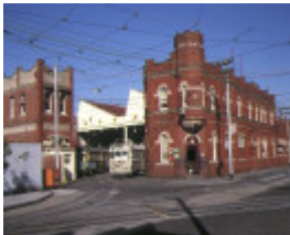
1 tram depot coldblo road malvern tram entrance
