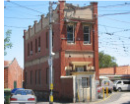
TRAM DEPOT SOHE 2008
