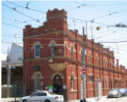
TRAM DEPOT SOHE 2008
