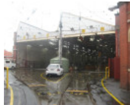
south car shed
