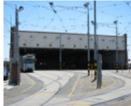
TRAM DEPOT SOHE 2008
