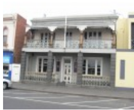
Wilkins House / Claredon Hotel (former), Hobsons Bay Heritage Study 2006
