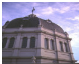
royal exhibition buildings nicholson street carlton dome detail
