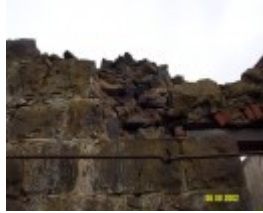
23113 Hilgay Coleraine detail of facade 1248
