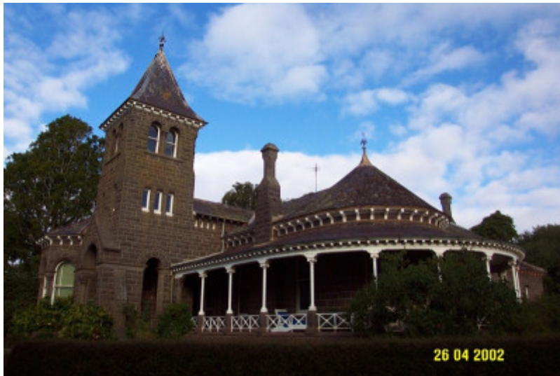
H0541 Kolor Penshurst entrance tower 0845
