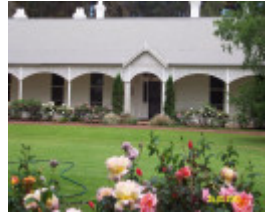
23195 Nareen Homestead Complex facade 1926
