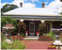
23233 Viladale House Yulecart facade 0308
