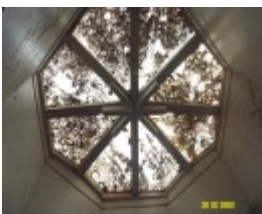
23435 Skene Homestead Strathkellar 1858 skylight 1613
