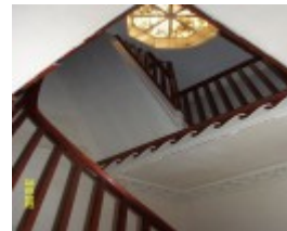
23435 Skene Homestead Strathkellar 1858 staircase 1605
