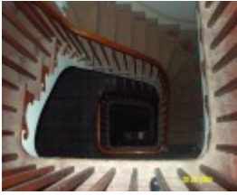
23435 Skene Homestead Strathkellar 1858 staircase 1615
