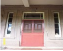
23435 Skene Homestead Strathkellar 1858 front door 1556
