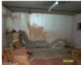
23435 Skene Homestead Strathkellar 1858 cellar 1589
