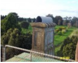
23435 Skene Homestead Strathkellar 1858 chimney 1612
