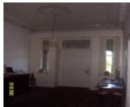
23435 Skene Homestead Strathkellar 1858 front door 1582
