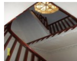
23435 Skene Homestead Strathkellar 1858 staircase 1605
