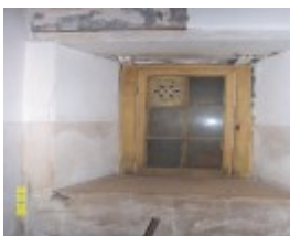
23435 Skene Homestead Strathkellar 1858 cellar 1598
