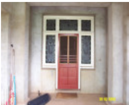
23435 Skene Homestead Strathkellar 1923 front door 1567
