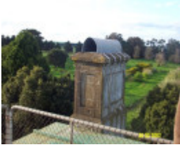
23435 Skene Homestead Strathkellar 1858 chimney 1612
