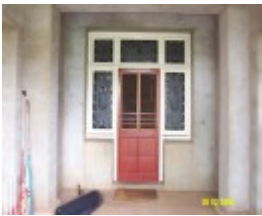
23435 Skene Homestead Strathkellar 1923 front door 1567
