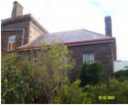
23435 Skene Homestead Strathkellar 1880s billiard room 1572
