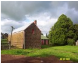
23435 Skene Homestead Strathkellar generator shed 1575
