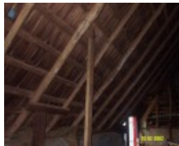
23435 Skene Homestead Strathkellar woolshed poles shingles 1635
