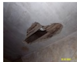
23435 Skene Homestead Strathkellar 1858 cellar 1595
