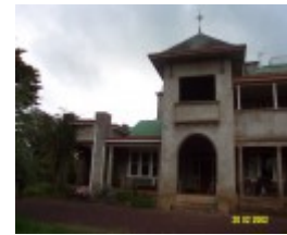
23435 Skene Homestead Strathkellar 1923 tower 1560
