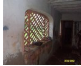
23435 Skene Homestead Strathkellar stables 1626
