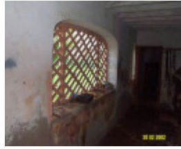
23435 Skene Homestead Strathkellar stables 1626
