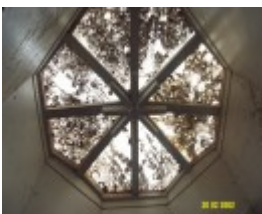
23435 Skene Homestead Strathkellar 1858 skylight 1613
