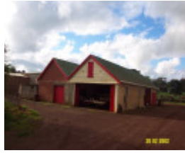
23435 Skene Homestead Strathkellar garages
