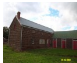
23435 Skene Homestead Strathkellar stables 1573
