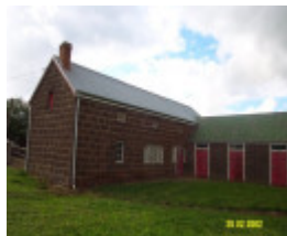
23435 Skene Homestead Strathkellar stables 1573
