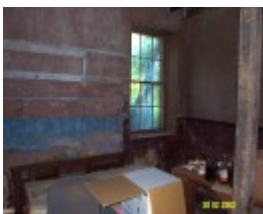
23435 Skene Homestead Strathkellar 1858 cellar 1593
