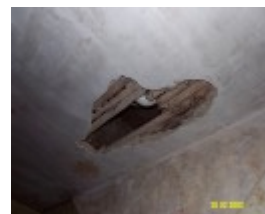
23435 Skene Homestead Strathkellar 1858 cellar 1595
