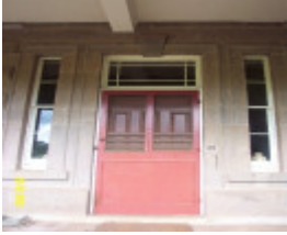
23435 Skene Homestead Strathkellar 1858 front door 1556
