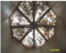
23435 Skene Homestead Strathkellar 1858 skylight 1613
