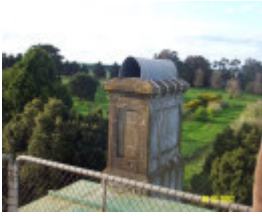
23435 Skene Homestead Strathkellar 1858 chimney 1612
