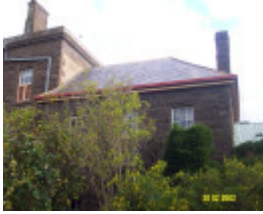
23435 Skene Homestead Strathkellar 1880s billiard room 1572
