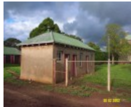
23435 Skene Homestead Strathkellar generator shed
