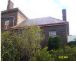
23435 Skene Homestead Strathkellar 1880s billiard room 1572
