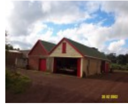
23435 Skene Homestead Strathkellar garages
