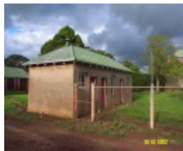
23435 Skene Homestead Strathkellar generator shed
