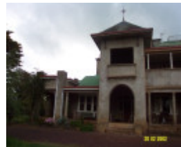
23435 Skene Homestead Strathkellar 1923 tower 1560
