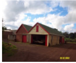
23435 Skene Homestead Strathkellar garages
