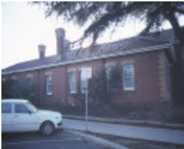
ararat court house side view jun1984
