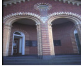
ararat court house entrance detail jun1984
