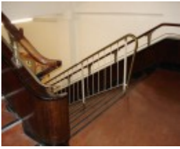
H2100 myers melbourne deco stairs 21 02 06 JB
