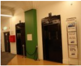
Myers Melbourne Elevators 5th Floor February 2006
