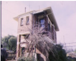
caulfield railway station normanby road caufield signal box aug1998
