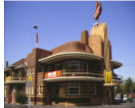
1 former united kingdom hotel queens parade clifton hill front view 1993
