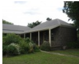
Correagh former kitchen wing
