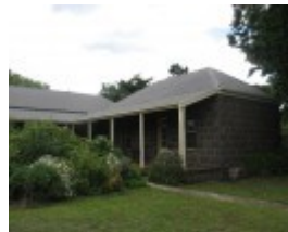
Correagh former kitchen wing
