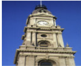
collingwood town hall clock tower detail jul1983
