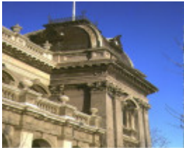
collingwood town hall balcony detail jul1983
