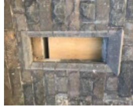
Repairs to B1
