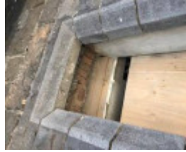
Repairs to B1
