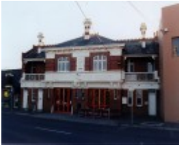
IVANHOE METROPOLITAN FIRE BRIGADE STATION
