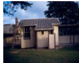
H02030 point nepean isolation hospital
