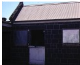
stables 1875 lara homestead derrinallum entrance
