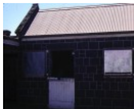
stables 1875 lara homestead derrinallum entrance
