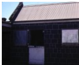
stables 1875 lara homestead derrinallum entrance
