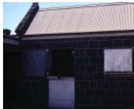
stables 1875 lara homestead derrinallum entrance
