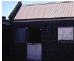
stables 1875 lara homestead derrinallum entrance
