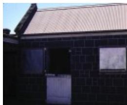
stables 1875 lara homestead derrinallum entrance
