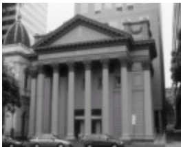
former baptist church house front elevation
