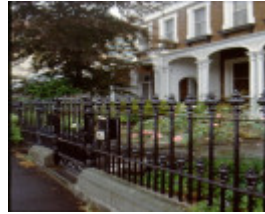
1 nepean terrace gipps street east melbourne facade january 2000
