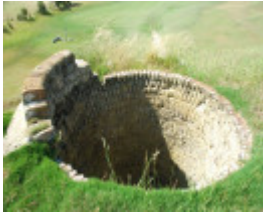
SULLIVAN'S LIME KILN SOHE 2008
