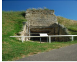
SULLIVAN'S LIME KILN SOHE 2008
