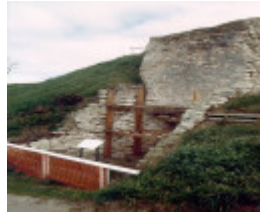
1 sullivan's lime kiln 2000
