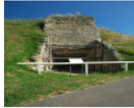
SULLIVAN'S LIME KILN SOHE 2008
