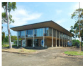
FORMER BP REFINERY ADMINISTRATION BUILDING SOHE 2008
