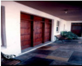
H01998 bruce manor frankston rear verandah
