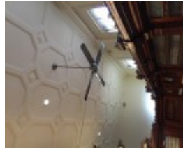
EASTERN HILL FIRE STATION July 2016
