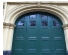
EASTERN HILL FIRE STATION July 2016
