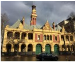
EASTERN HILL FIRE STATION July 2016
