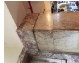
EASTERN HILL FIRE STATION July 2016
