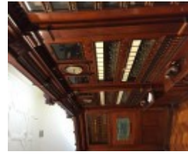
EASTERN HILL FIRE STATION July 2016
