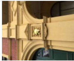
EASTERN HILL FIRE STATION July 2016
