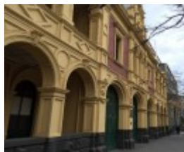
EASTERN HILL FIRE STATION July 2016
