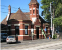
FORMER RICHMOND SOUTH POST OFFICE SOHE 2008
