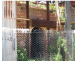
WUNDERLICH/MONIER TERRACOTTA ROOF TILES COMPLEX SOHE 2008
