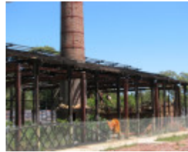
WUNDERLICH/MONIER TERRACOTTA ROOF TILES COMPLEX SOHE 2008
