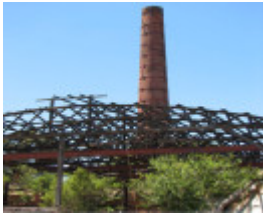
WUNDERLICH/MONIER TERRACOTTA ROOF TILES COMPLEX SOHE 2008
