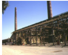
1 wunderlich terra cotta tile works demolished mitcam road vermont view of chimneys nov1993
