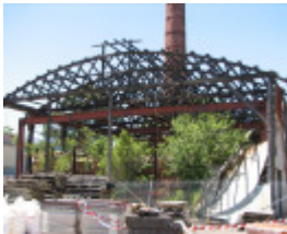
WUNDERLICH/MONIER TERRACOTTA ROOF TILES COMPLEX SOHE 2008
