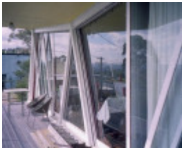
h01906 mccraith house atunga terrace dromana verandah she project 2003
