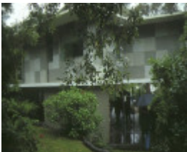
Delbridge House Eaglemont Rear View 1995
